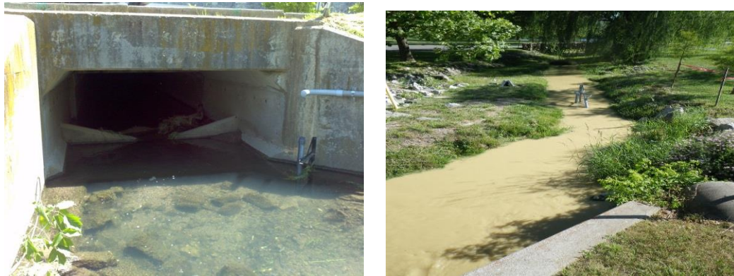
Figure 2: LEWAS Site during normal flow and during the water main break
