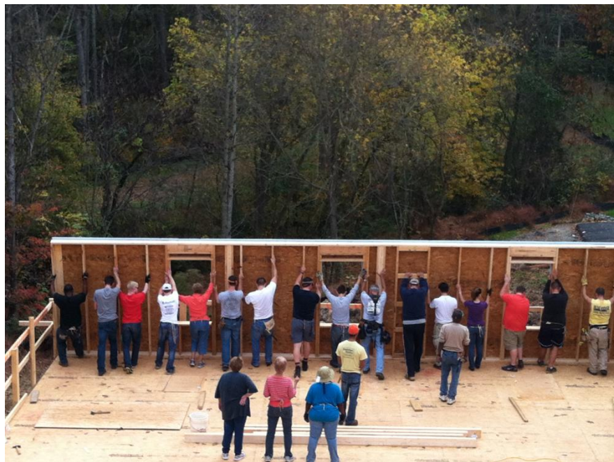
Figure 1. HFH Participating Students Erecting Framing Wall
