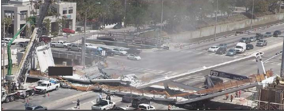
Figure 2. View of the collapsed FIU pedestrian bridge on March 15, 2018 (from [11])
