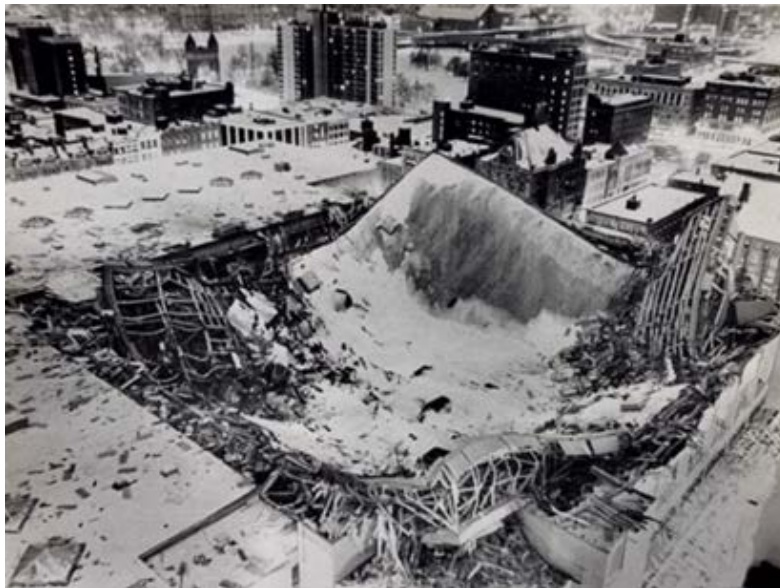
Figure 1. View of the Hartford Civic Center roof, January 1978 – Connecticut Historical Society (from [8])
