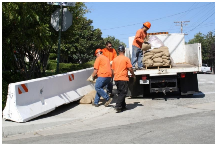
Figure 2. K-Rail being installed in La Crescenta, CA. Photo courtesy of Crescenta Valley Weekly.
