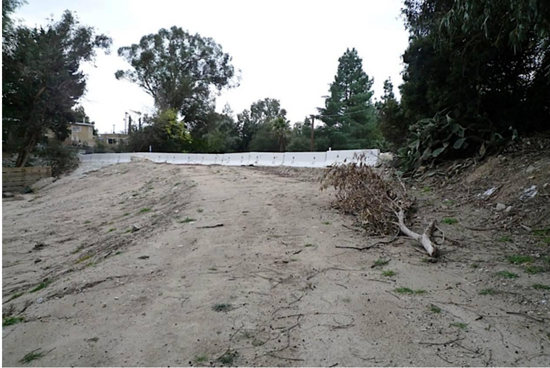
Figure 3. Line of K-Rails installed in Rosemont Preserve. Photo courtesy of Tim Wendler and Paul Rabinov.
